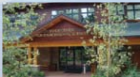
GREEN BUILDING TOURS
